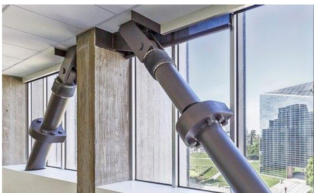
Figure 2 Fluid Dampers as bracing element
