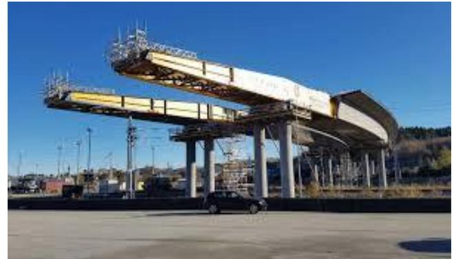
Figure 1 Incremental Launching Method
