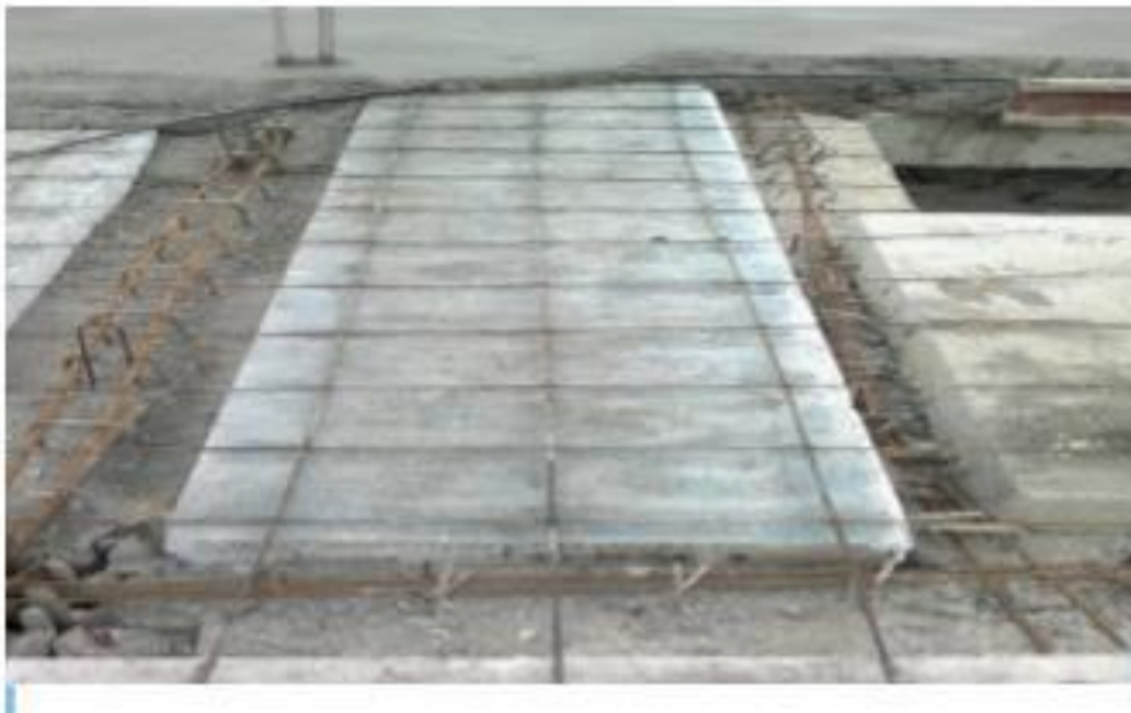
Figure 4.12 Sample of Prefabricated Siporex Slab
