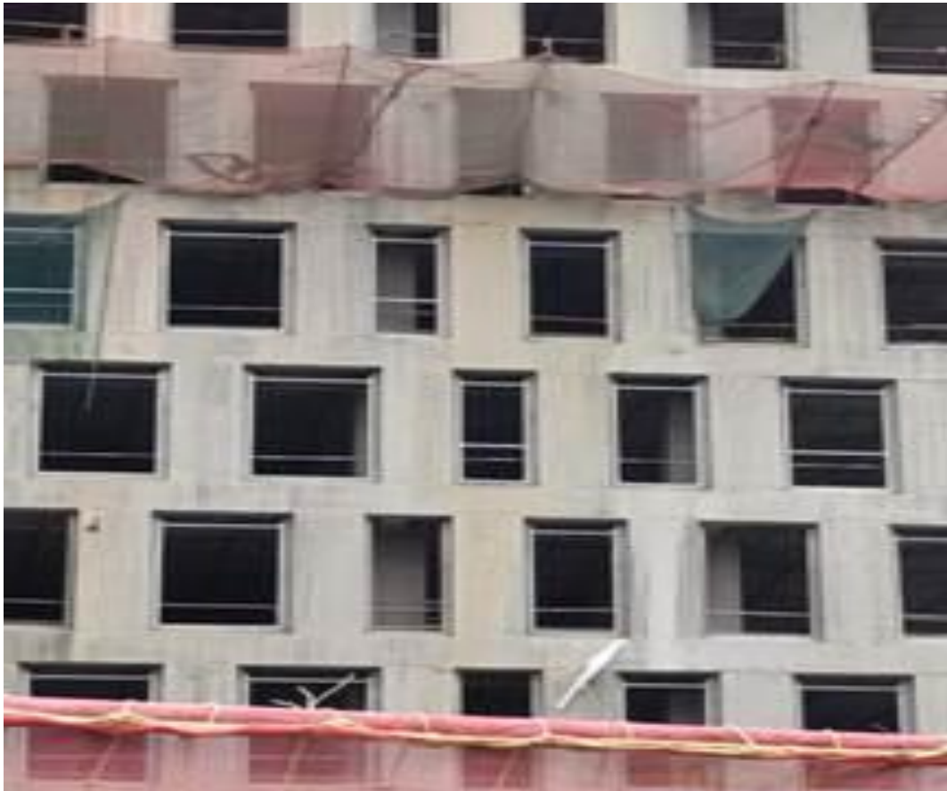
Figure 4.3 buildings under construction
