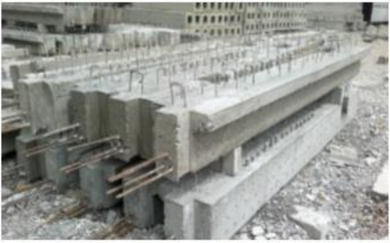
Figure 4.8 Sample of Prefabricated Beam
