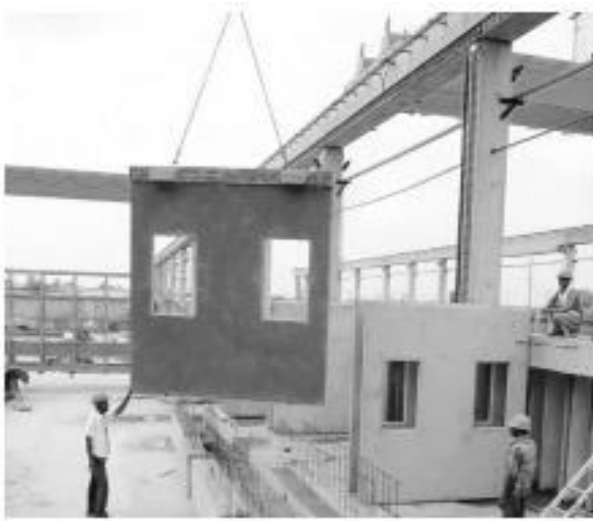
Figure 4.14 Precast wall panels
