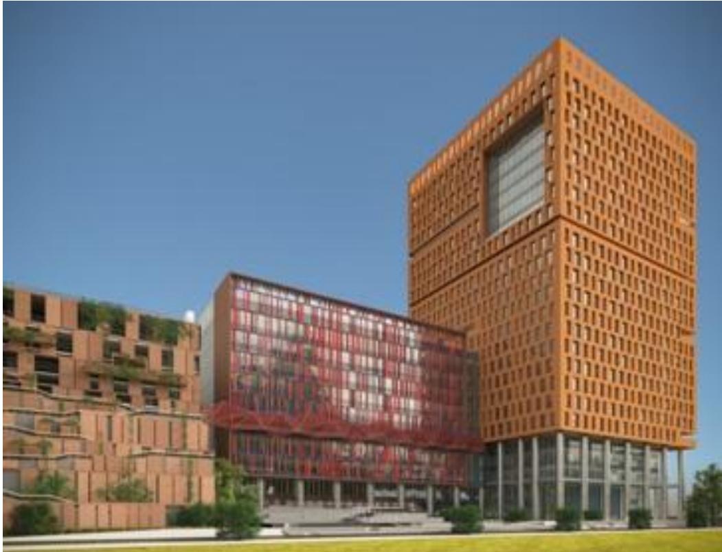
Figure 4.1 IT Park comprising of 3 buildings B9, B10 & B11 consists
