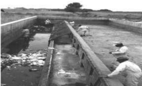
Fig.1: View of an SCS litter trap (near Springs, South Africa) being cleaned and repaired
